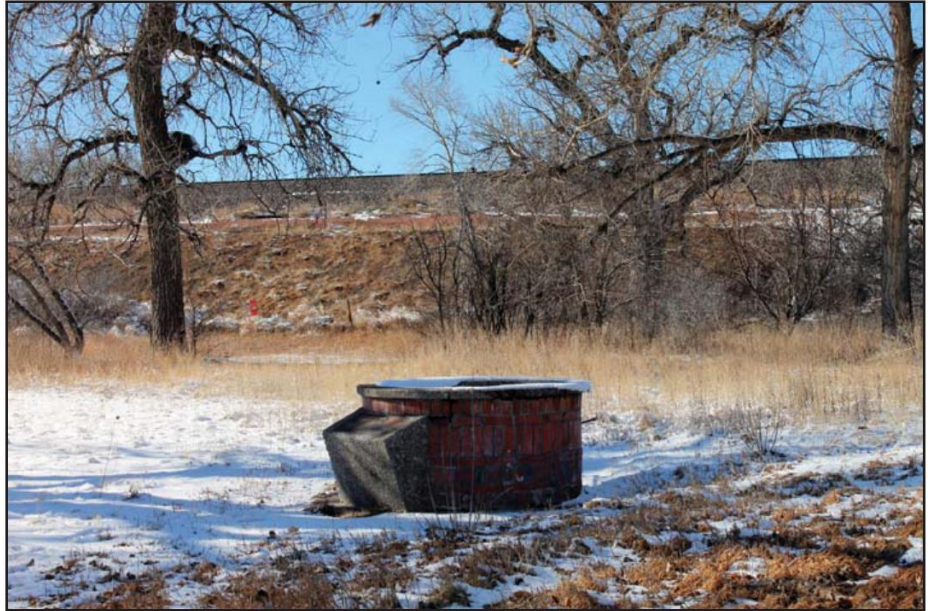
The well at Church's Stage Stop located at 10395 Wadsworth Boulevard. Photograph taken facing west, January 28, 2014.
