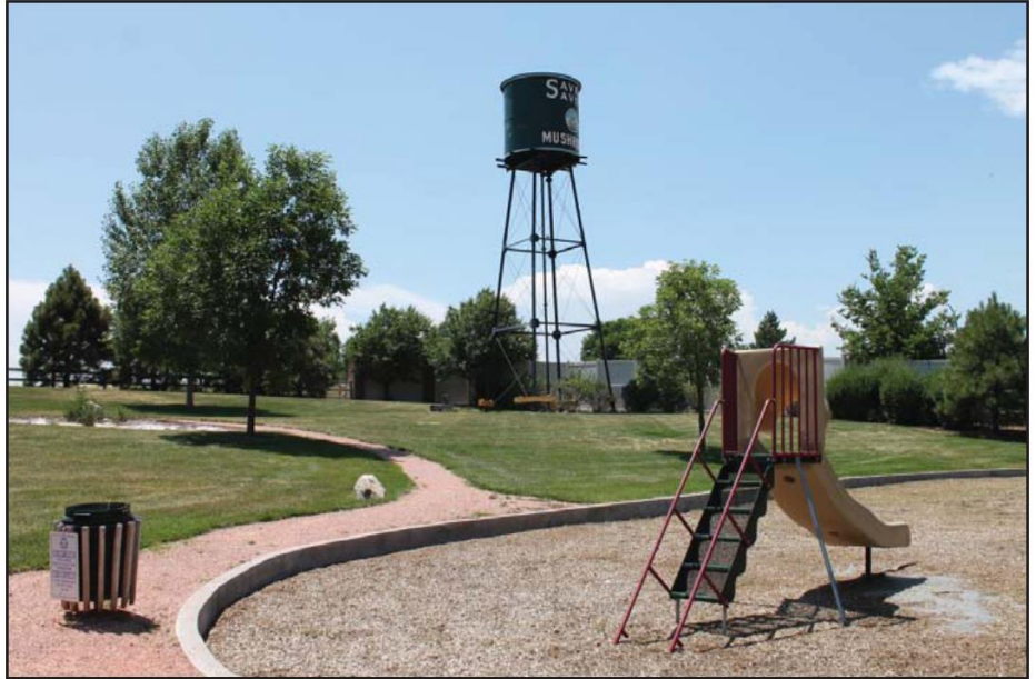
Savery Savory Mushroom water tower is the only remaining structure of the Savery Savory Mushroom Farm. Photograph taken facing south towards Federal Boulevard, July 3, 2014.
