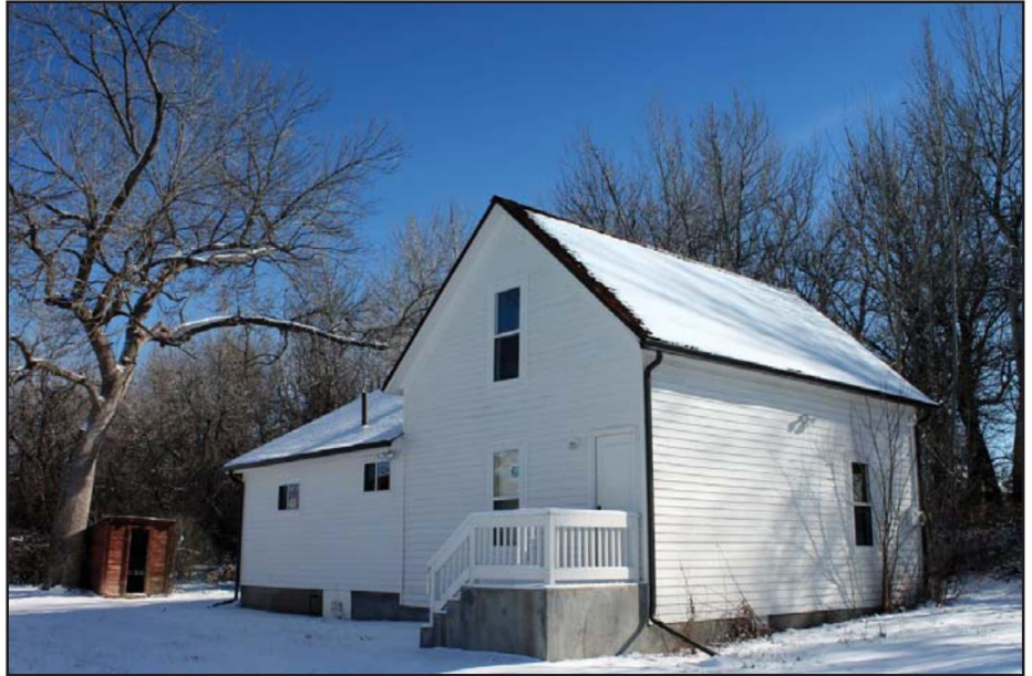
The main residence at the Charles and Julia Semper Farm, also known as the Allison Farm, located north of West 92nd Avenue on the east side of Pierce Street. Photograph taken facing southeast, January 28, 2014.
