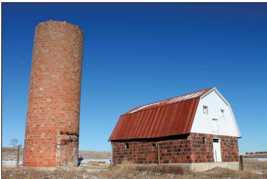
The barn and clay-tile silo at the Tucker Ranch/Lower Church Lake, located on the east side of West 108th Avenue and Wadsworth Boulevard. Photograph taken facing northeast, January 28, 2014.
